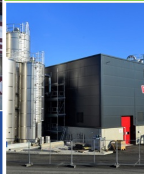
Industrial Applications & District Heating
