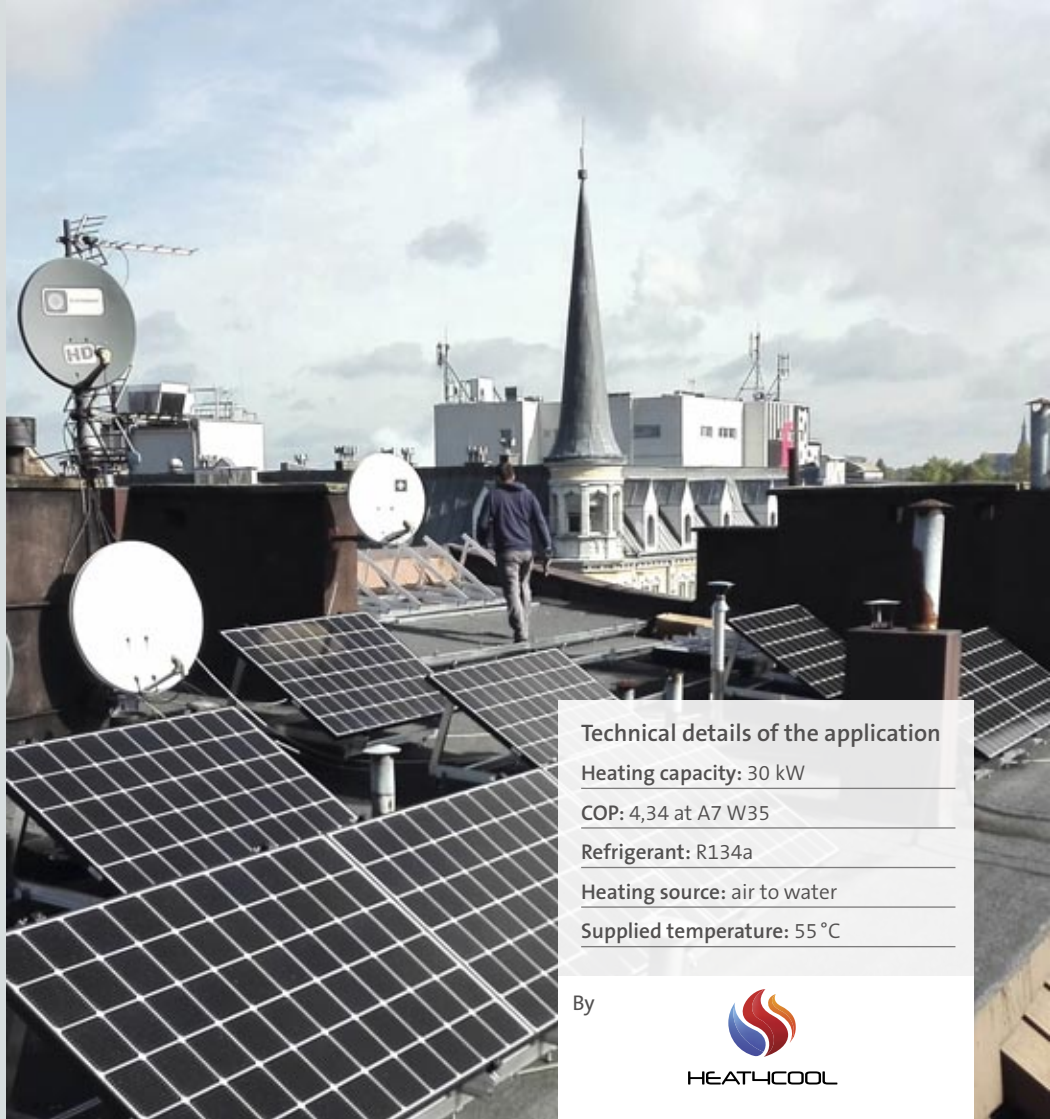
Picture 3 (right): PV modules installed on the roof Source: Heat4Cool project
