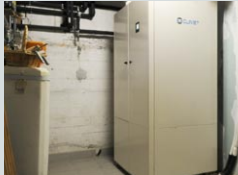
Picture 3 & 4: Clivet heat pump installed in the technical room instead of old boiler and tank
