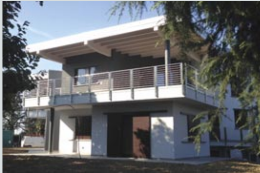
Picture 1 & 2: Single-family house before and after requalification
