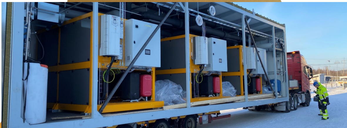
The system consists of three Calefa high-temperature heat pumps with total heating power of 1,5 MW.
