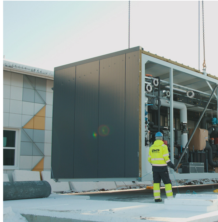
Factory-installed and factory tested heat pump plant modules being delivered to the site.
