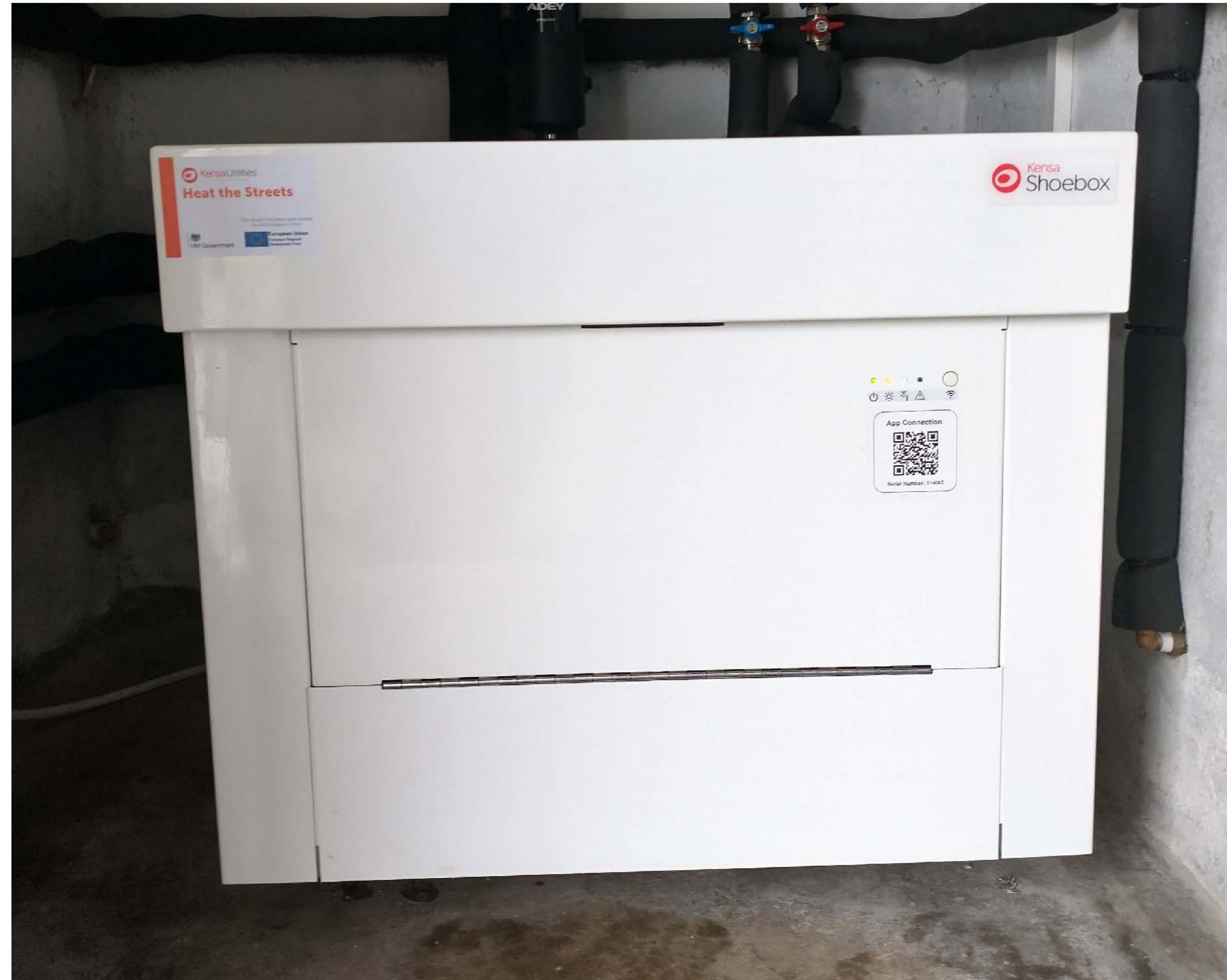
The Kensa Shoebox heat pump, roughly the size of a microwave - Copyright Kensa Utilities
