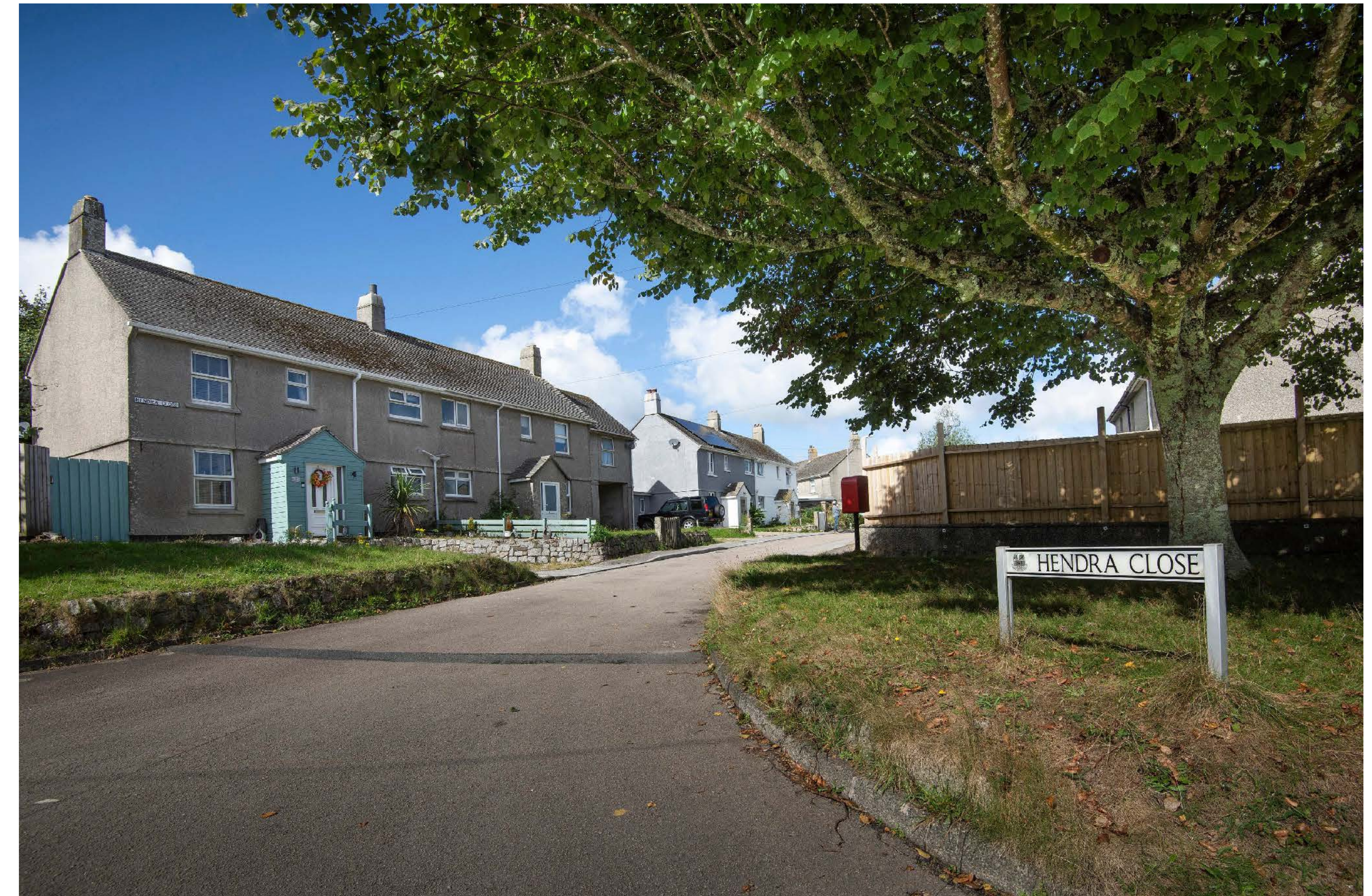
Hendra Close - Copyright Kensa Utilities
